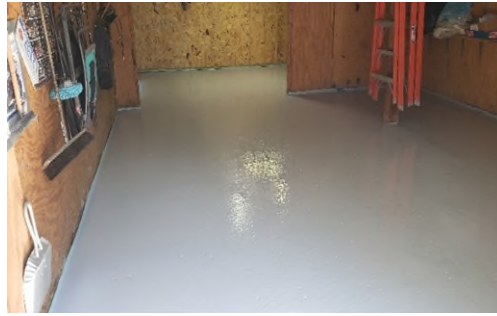
34380 Beacon garage RetroCoat
