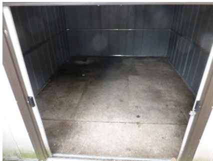
34401 Capitol shed before
