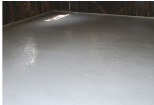
12066 Boston Post garage RetroCoat
