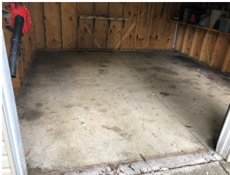
34380 Beacon shed before
