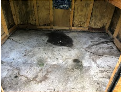
34424 Beacon shed before
