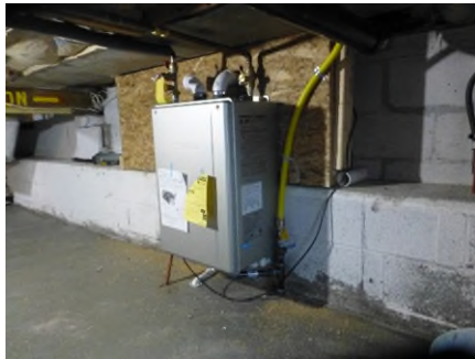
12070 Boston Post tankless water heater
