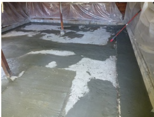
12089 Boston Post garage concrete repair
