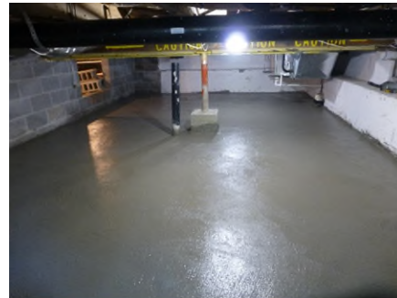
12070 Boston Post sump in new floor slab
