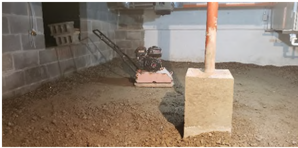
12070 Boston Post gravel fill
