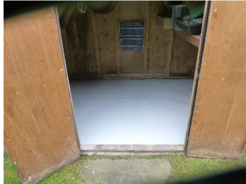
34424 Beacon shed RetroCoat
