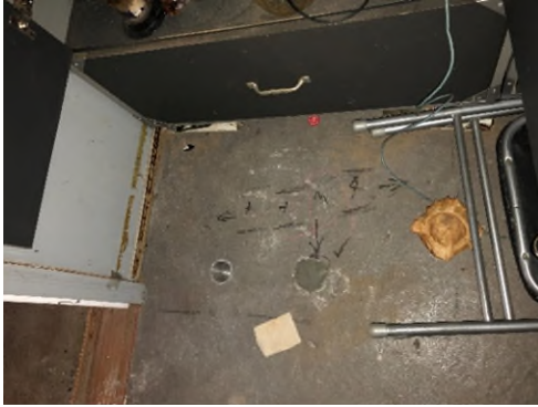
12101 Brewster replaced monitoring point
