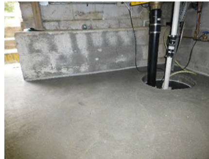
12070 Boston Post sump in new floor slab
