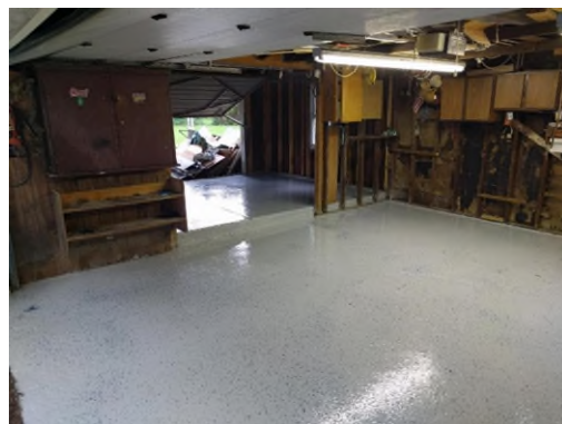
12067 Boston Post garage RetroCoat
