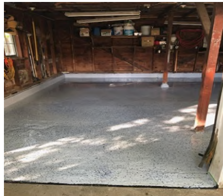
12089 Boston Post garage RetroCoat
