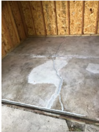
12036 Brewster shed before
