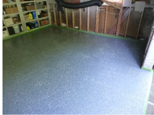
12101 Brewster garage epoxy coating
