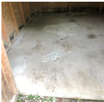
12075 Brewster shed before
