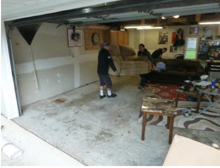
34480 Capitol garage before
