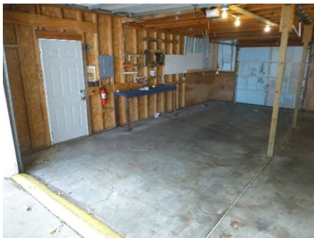
34367 Capitol garage before
