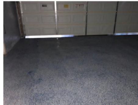
34920 Beacon garage RetroCoat
