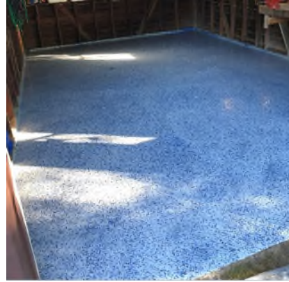
34950 Beacon garage RetroCoat
