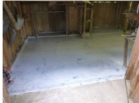
12131 Boston Post garage RetroCoat
