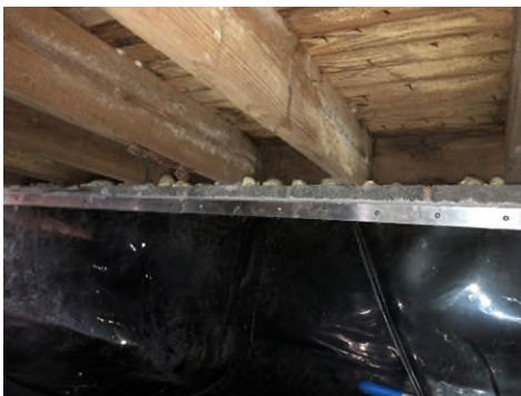
34424 Capitol barrier installation
