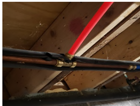
34424 Capitol plumbing repair
