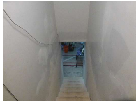
34990 Beacon installed stairwell
