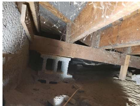
12124 Boston Post structural support, inaccessible space
