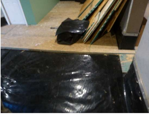
12131 Boston Post plywood flooring removed for moisture investigation
