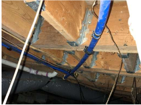
34450 Capitol water lines replaced for access
