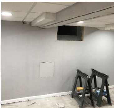
34990 Beacon installed drywall with access panel
