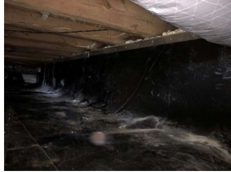
34450 Capitol installed and battened barrier
