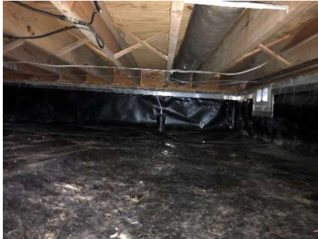
34644 Beacon installed barrier and monitoring point
