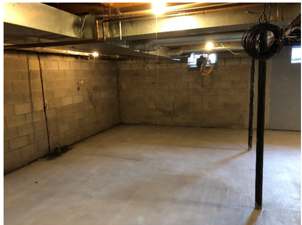
Completed concrete floor with RetroCoat™ primer on the walls
