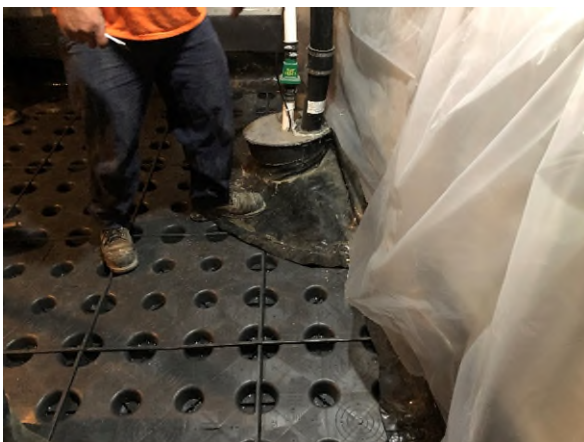
Cupolex flooring and sump prior to concrete pour
