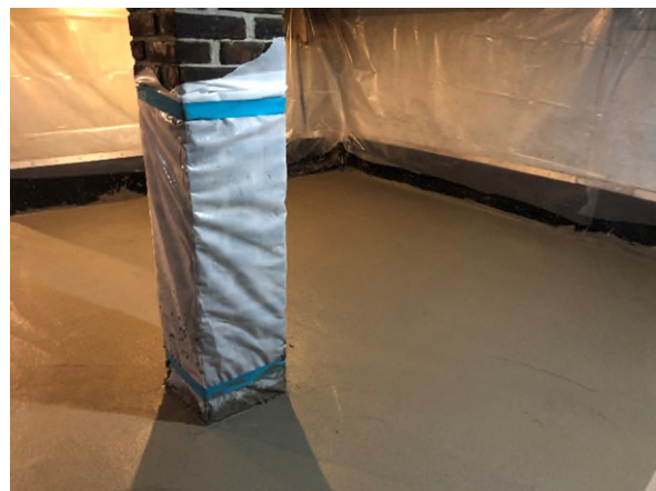
Newly poured concrete floor
