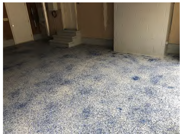
Retro-coat applied to the concrete floor in the garage.
