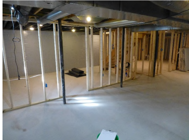
Rebuild of the finished walls in the basement.
