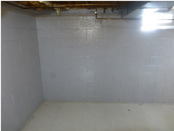
Finished concrete pour, and retro-coat applied to the basement walls.
